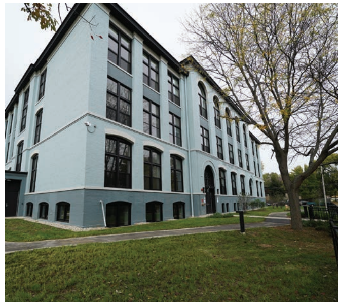
One of the Foundation's campaign goals is to bring safe, affordable housing within reach of all. Pictured is the former 37th Street School near Washington Park, an affordable housing development featuring 49 units for adults 55 years and older.
